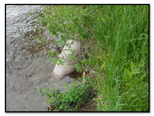
Figure 5: 20SA722, eroded well casing.
